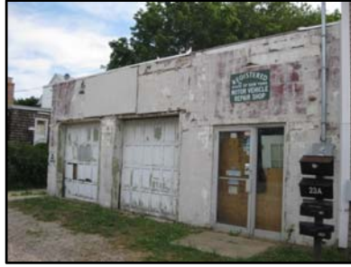
Photograph 1: View of deteriorated building along the east side of Hawkins Avenue.
